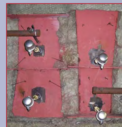
Installation of McOn air in power station
