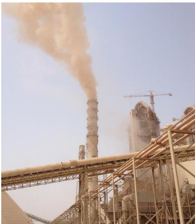
Broken bag filter, which can be monitored and recorded.
