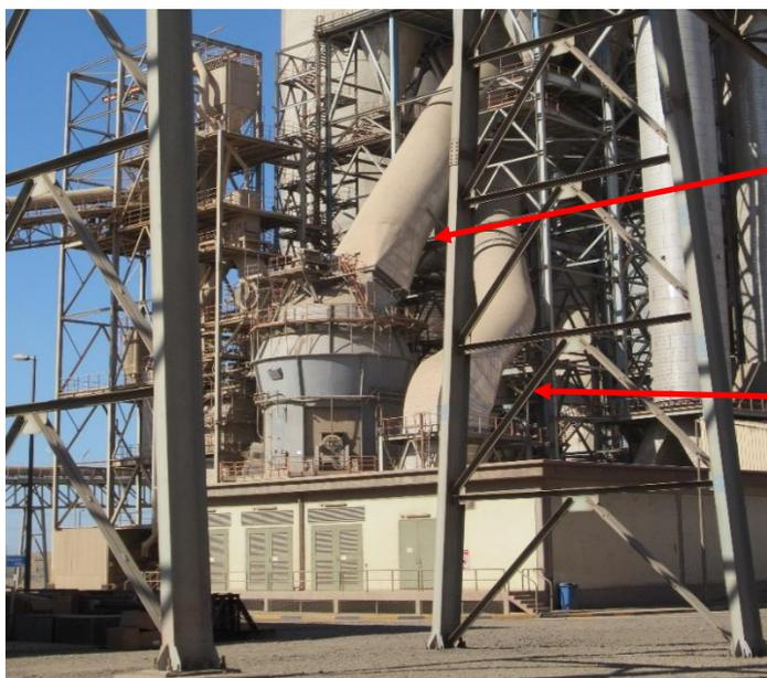
Material flow / gas flow out of the mill
