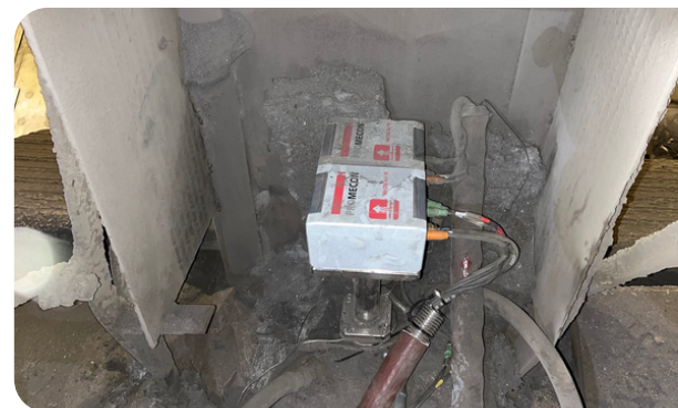
Installation situation at FERALPI STAHL in Riesa
